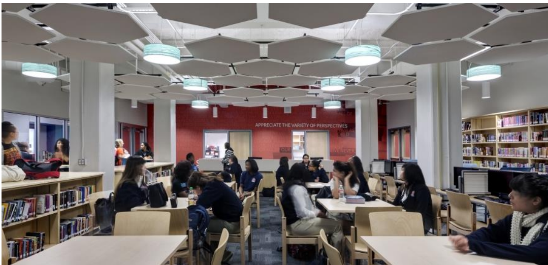
Young Women's Leadership Academy LMC, Fort Worth, Texas (Design by Perkins+Will) Open acoustical ceiling panels provide sound absorption while allowing the sense of higher ceiling above.
