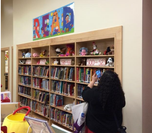
Red Pump Elementary School LMC, Bel Air, MD (Designed by GWWO) Inset shelving in the wall is an option to create a cleaner look and to ensure the shelving is out of the way of other functions and circulation.
